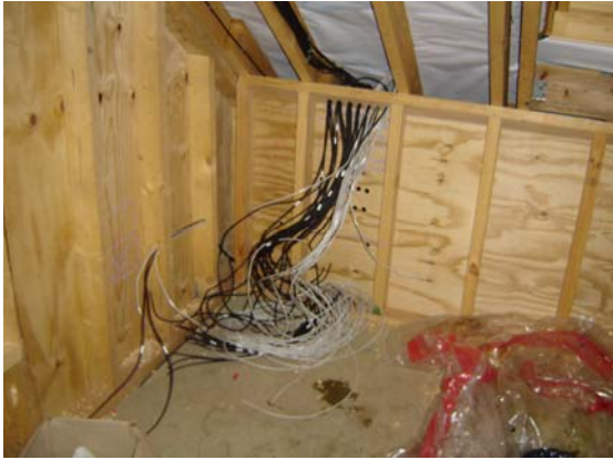
First fix cabling, making sure to label everything!
