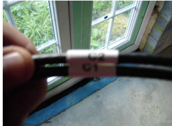
First fix cabling, making sure to label everything!
