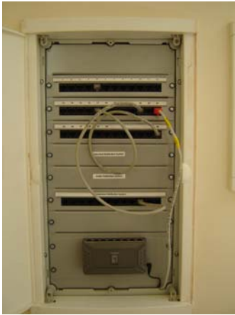
The result of second fix in the hub room – neat, flush mounted with everything behind closed doors!
