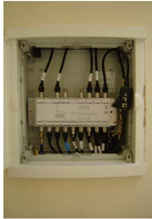
The result of second fix in the hub room – neat, flush mounted with everything behind closed doors!
