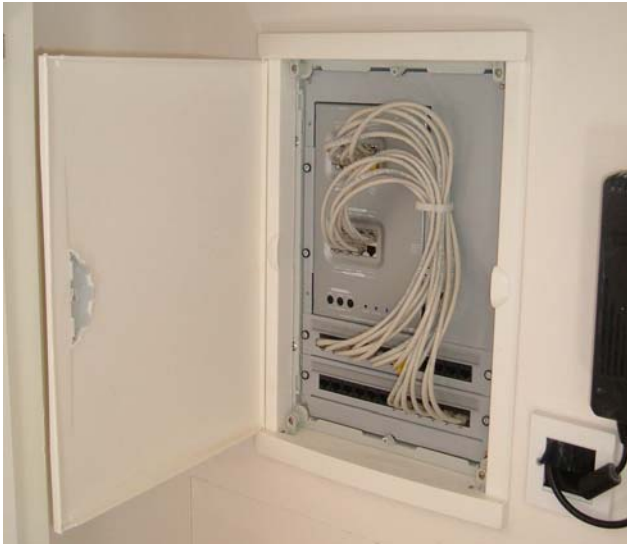
Upstairs...the central hub for the AV, TV, phone and broadband network
