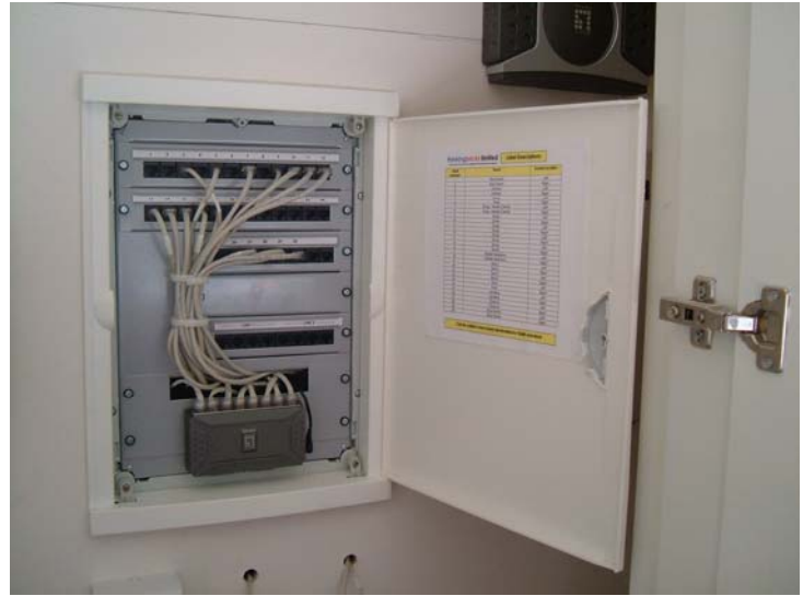
Upstairs...the central hub for the AV, TV, phone and broadband network
