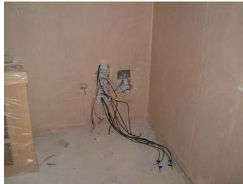
Day One – first fix cabling in place
