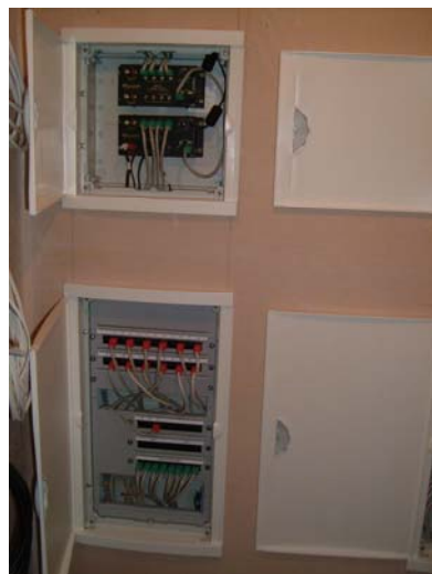
The Hub Room - TV and broadband on one side, audio and telephone on the other – neatly finished!
