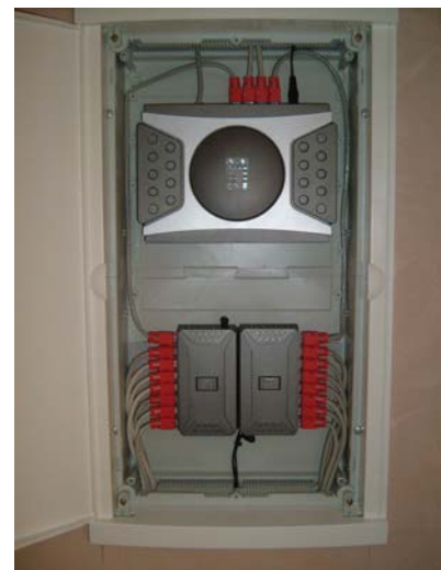
The Hub Room - TV and broadband on one side, audio and telephone on the other – neatly finished!
