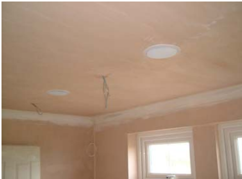
Second fix - speakers in, CAT5 terminated, keypads connected
