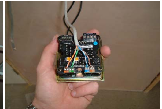
Second fix - speakers in, CAT5 terminated, keypads connected
