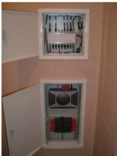
The Hub Room - TV and broadband on one side, audio and telephone on the other – neatly finished!
