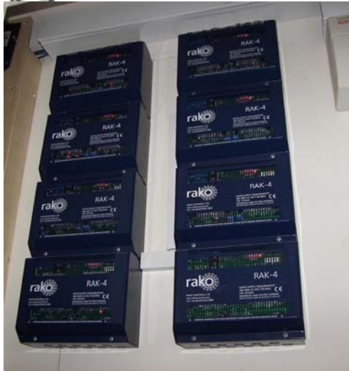
Behind the scenes – Rako lighting control racks and the Living control audio server and central controller – neat and tidy
