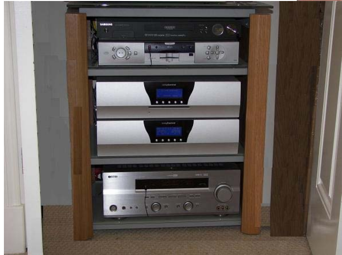
Behind the scenes – Rako lighting control racks and the Living control audio server and central controller – neat and tidy
